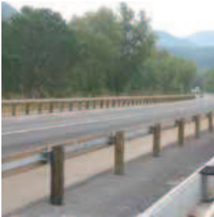
Half round log diameter 22 cm, length 4.00 m or 2.00 m backed with a steel U profile.
